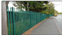
Proposed Fencing New boundary fencing to match existing along Ewerle Road 2.1m High Green powder-coated galvanized fencing
